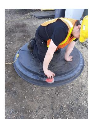
Wipe down the surface of the inner bead on the tank with Methyl Hydrate twice to make it as clean as possible. Sand the underside of the plug where it will meet the tank and the urethane adhesive. After sanding, wipe the plug clean then apply a 2" strip of the adhesive primer all around the plug in the area where it will sit on the adhesive. Apply 2 coats of primer about 20 minutes apart. Allow 20 minutes to dry apply final coat.
